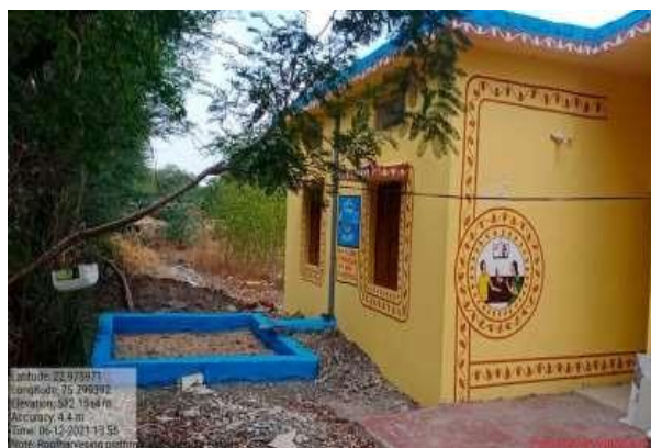
Rain water harvesting structure constructed as part of the "catch the rain" campaign at GP building in MP
